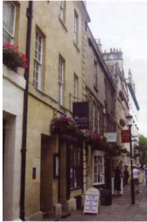
Above: (left) the north and (right) south elevations of No.2 North Parade Passage.
